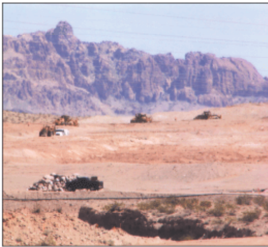
Heavy equipment vehicles from R.E. Monk Construction Co. of Fountain Hills, Ariz. – being operated 21 hours per day, 7 days per week – have moved nearly 4,000,000 cubic yards of earth for state-of-the-art Laughlin Ranch Golf Club toward north end of the Bullhead Parkway. Par-72 championship golf is expected to be completed and in operation in late December. (Photo by Ron Morrison)
